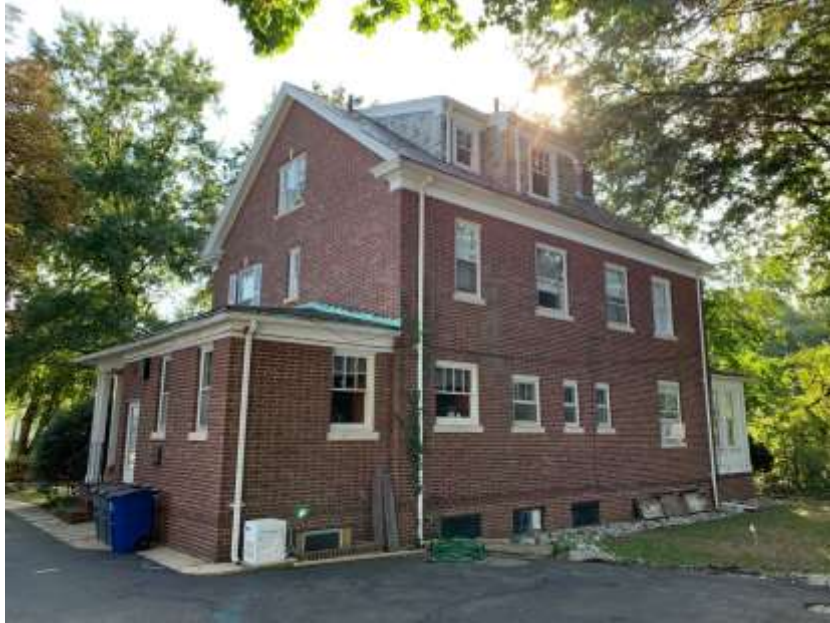
Figure 3: View of house from backyard; showing height of building
