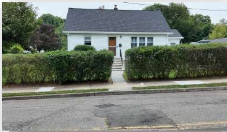
Figure 3. 201 Walnut across from the subject site.
