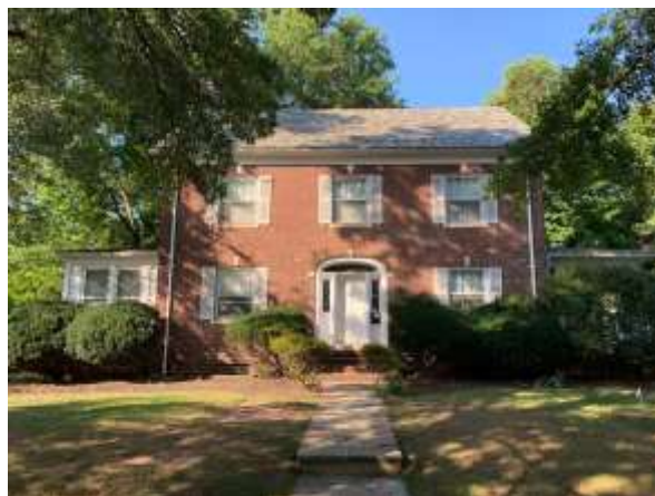
Figure 2: Looking toward the front of the property from Hazelwood Road
