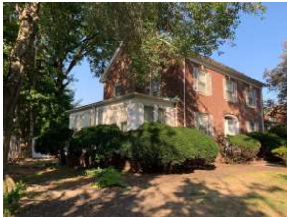
Figure 1: Looking towards property on the corner of Hazelwood Road and Walnut Avenue
